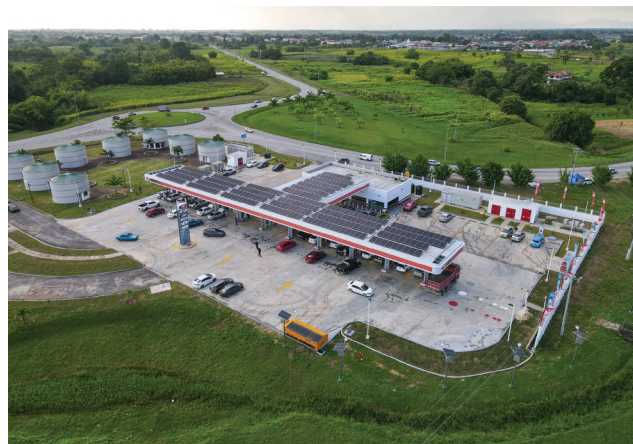
Figure 1: 320 South Facing Solar panels at the Preysal Service station which forms part of the PV System.
